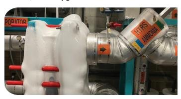
As part of its commitment to energy efficiency and visitor comfort, WSPRS upgraded the aging refrigeration system at the Q Centre Arena. The previous shell and-tube chiller was replaced with a modern, energy-efficient plate-and-frame chiller. The new system offers a smaller footprint, lower energy use due to its faster heat transfer, easier maintenance with replaceable parts, and future expansion potential. It also requires less ammonia, reducing risk and improving safety.
